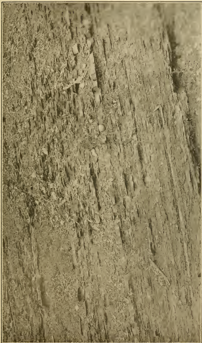
PLATE LXXII.—A typical exposure of Portage Shale and Sandstone at Mathias in the southeastern part of the county. The exposure shows about 35 per cent. sandstone and 65 per cent. shale. The sandstone layers are from about 2 inches to about 10 inches in thickness. The Portage is practically without fossils.
